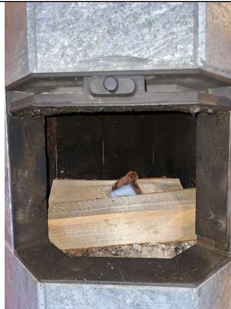
Step 2: Put bark and igniting bag in between logs.
