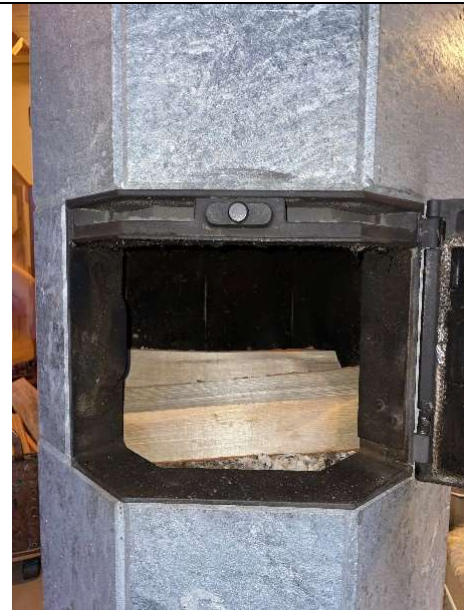
Step 1: Put in 2 larger logs close together.
